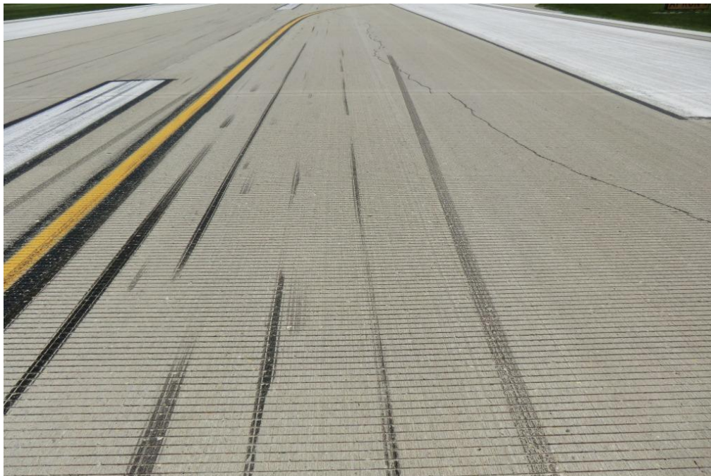
MKT RY1533 002 (Low-Severity LTD Cracking)
