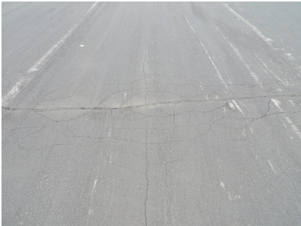
MKT TLE 001 (Alligator Cracking)
