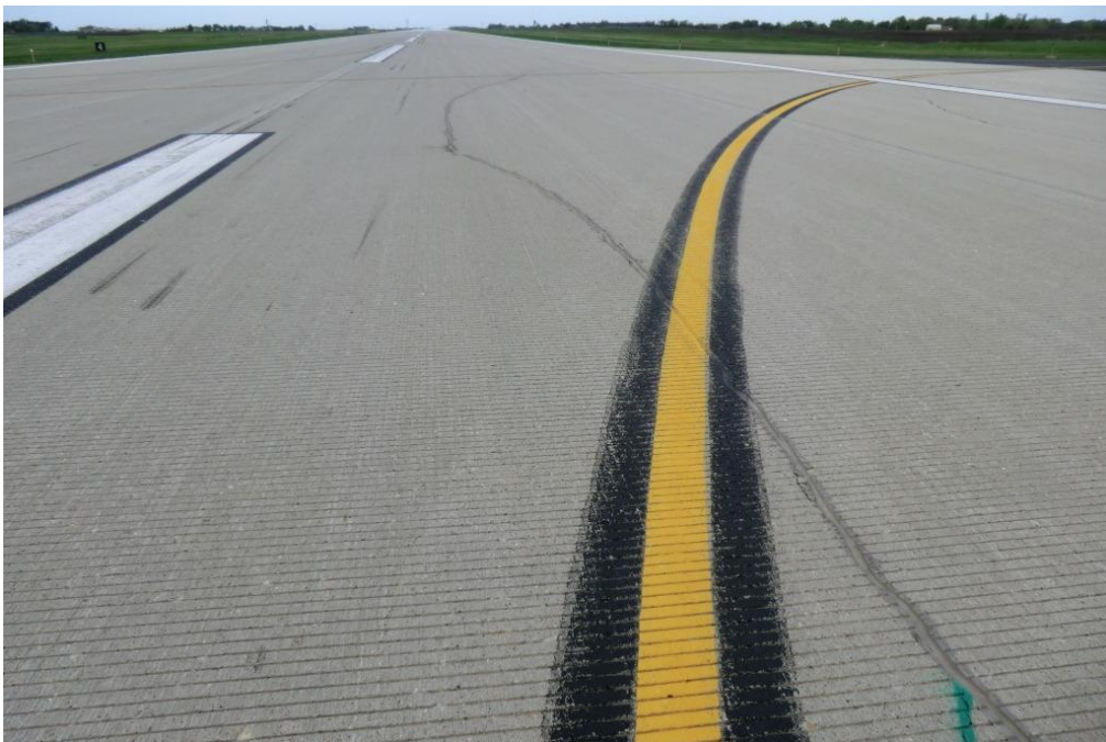
MKT RY1533 001 (Low-Severity LTD Cracking)
